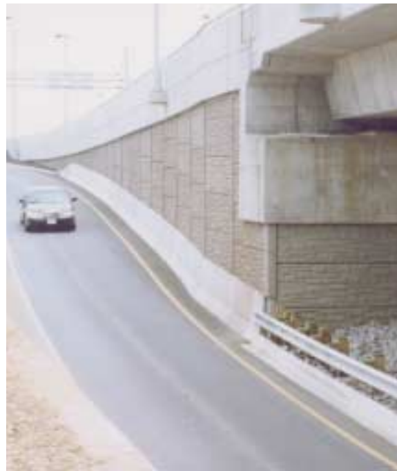
Lester B. Pearson International Airport - Toronto, Ontario False Abutment MSE Retaining Wall incorporating lower retaining precast traffic barrier and upper precast traffic barrier
