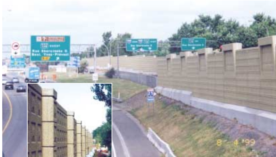
Auto Route 25 - City of Montreal, MTQ Custom Architectural Noise Wall Panels & Post Cladding
