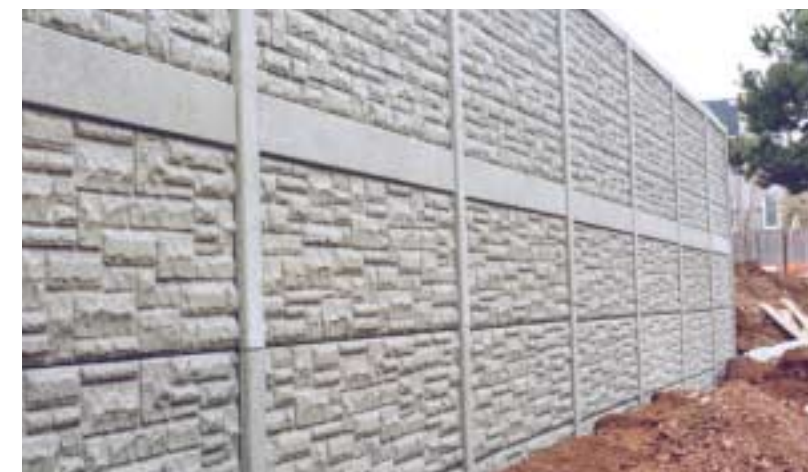
Burger King - Oakville, Ontario Durisol MSE type Retaining Wall with Noise Barrier.
