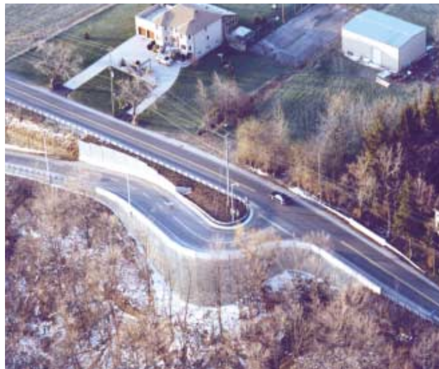
Lester B. Pearson International Airport - Toronto, Ontario False Abutment MSE Retaining Wall incorporating lower retaining precast traffic barrier and upper precast traffic barrier
