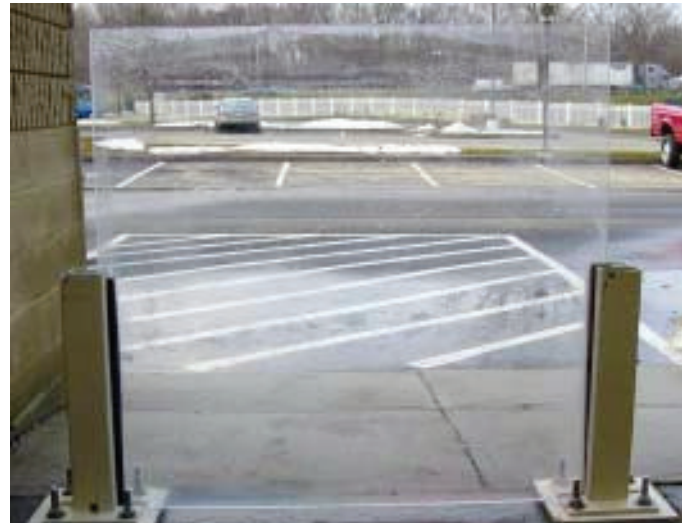
4. AFTER WATER RINSE WITH 2,300PSI PRESSURE WASHER
