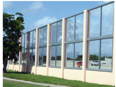
MIAMI, FL - (ALUMINUM) READY-FIT FRAMES INSTALLATION
