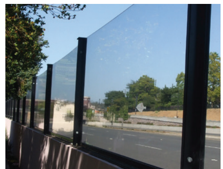
FOLSOM, CA - ACRYLITE® SOUNDSTOP NOISE BARRIER PANELS
