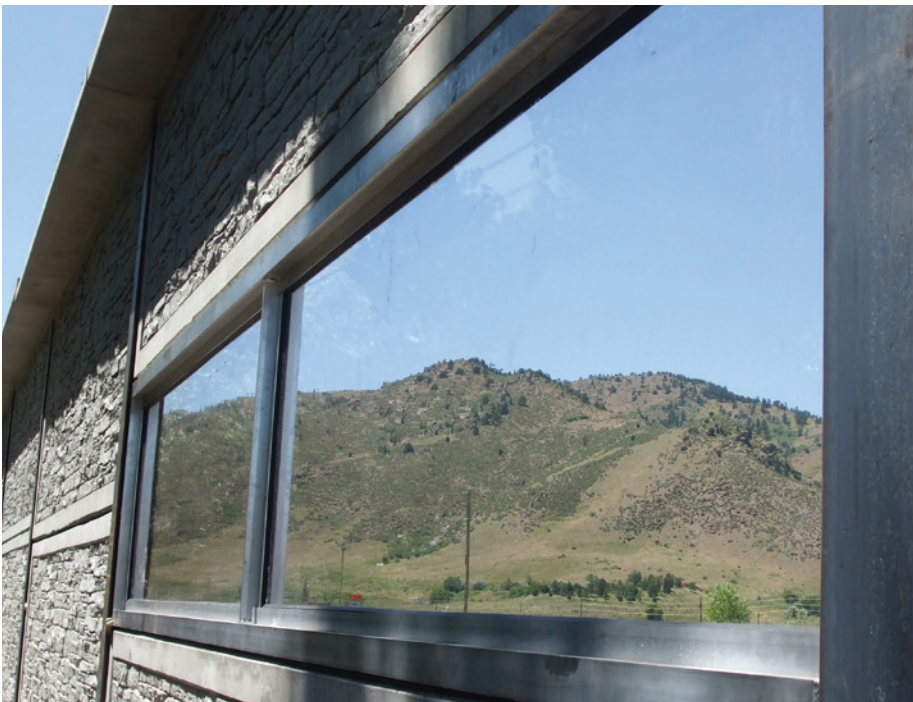
GOLDEN, CO - ACRYLITE® SOUNDSTOP NOISE BARRIER PANELS
