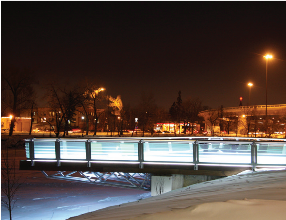
CALGARY, AB - ACRYLITE® SOUNDSTOP NOISE BARRIER PANELS
