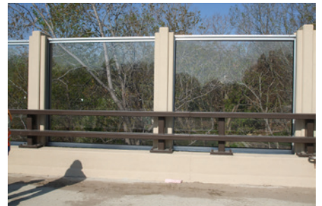
CROSTOWN, MN - ACRYLITE® SOUNDSTOP NOISE BARRIER PANELS
