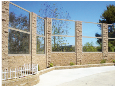
LAGUNA HILLS, CA - ACRYLITE® SOUNDSTOP NOISE BARRIER PANELS
