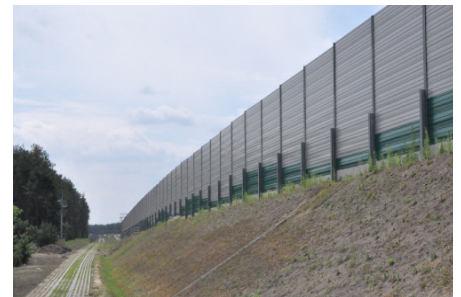
REAR-VIEW OF HIGHWAY BARRIER
