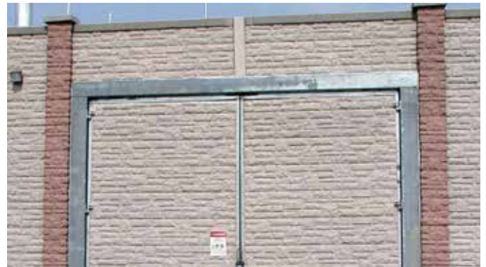
VEHICLE ACCESS GATE
