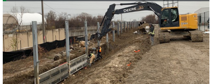
Installation of lower MSE earth retaining wall panels
