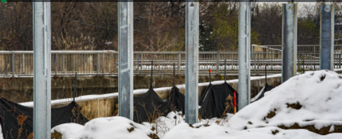
Combination Noise & Earth Retaining wall posts installed
