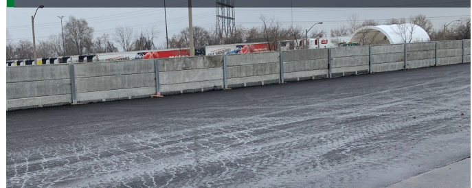
Completed wall installation
