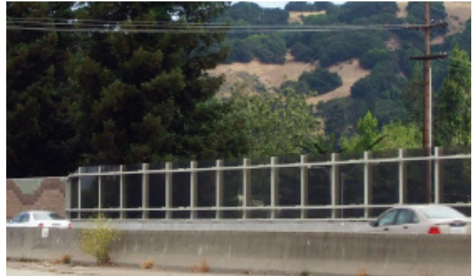
INTERSTATE 580 - SAN LEANDRO CA
