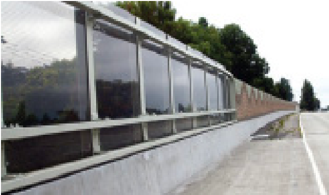
INTERSTATE 580 - SAN LEANDRO CA
