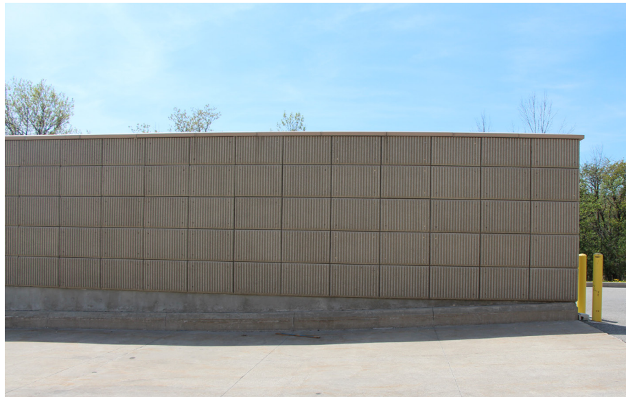
WALMART LOADING AREA, MARKHAM, ON
