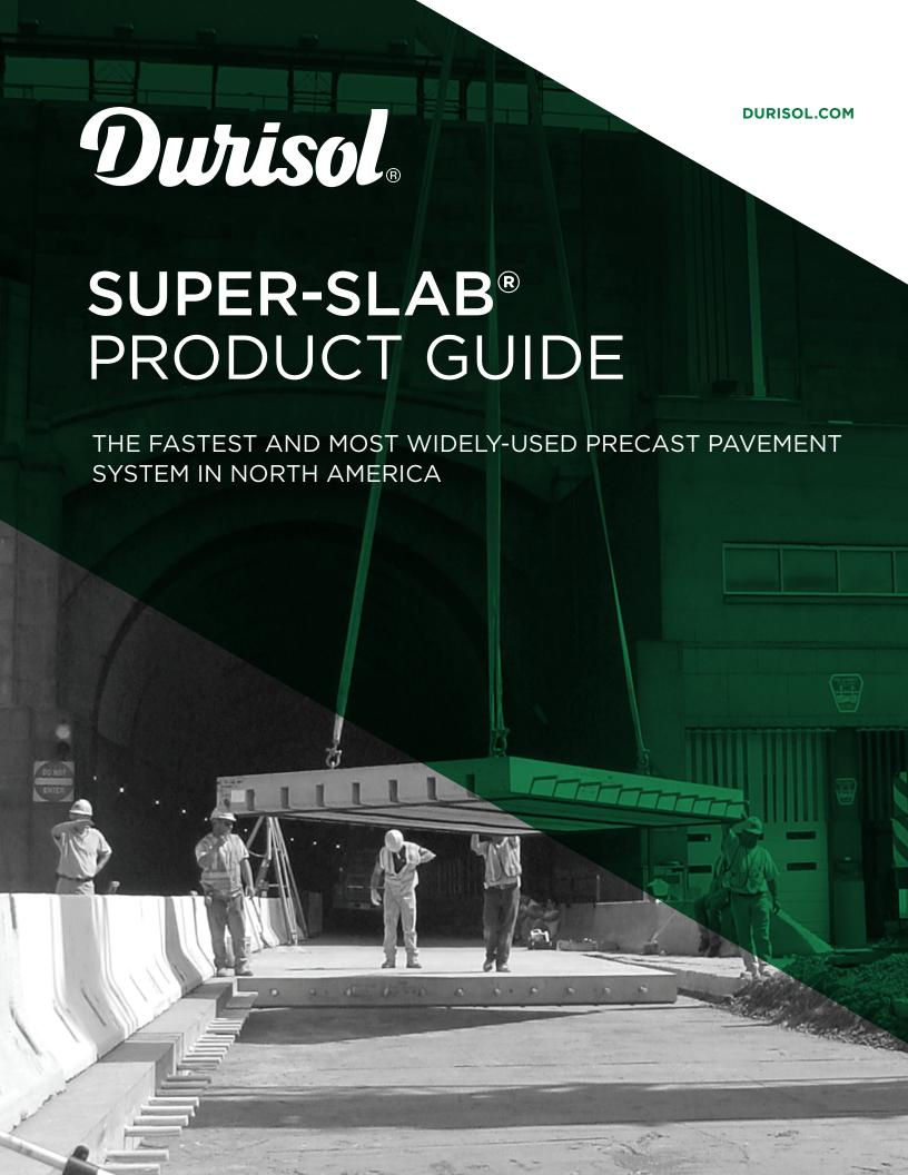
The Super-Slab® System places precast slabs directly upon a fully engineered sub-grade surface that provides nearly complete slab support immediately upon installation. After the slabs have been placed, they are structurally interlocked with a unique grouted load transfer system. Complete slab support is achieved when bedding grout is pumped into a bedding grout distribution system that is cast into the bottom of the slabs.
